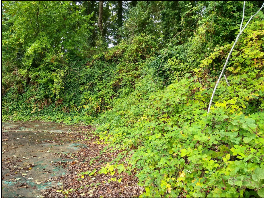
Photo 3. Steep cut-slope excavated to create the terrace.
