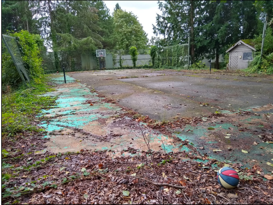
Photo 1. Tennis court occupies much of the property area.
